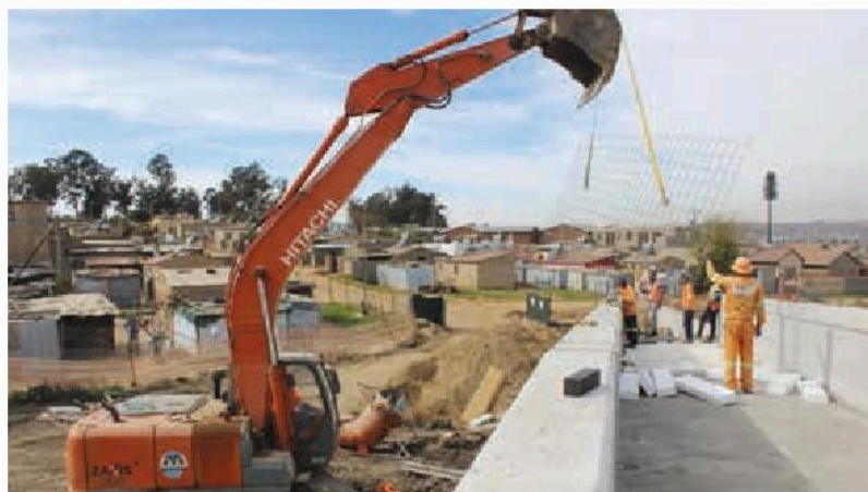
The hollow-core slabs are first covered with polystyrene moulds with voids to reduce the load of the 150 mm-thick final concrete slab on the precast-concrete beams. Services are then installed on top of the polystyrene moulds and covered with a steel mesh to reinforce the slab.
