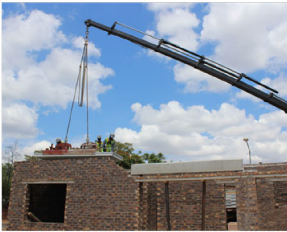
The hollow-core slabs were placed in a matter of a few hours by CoreSlab’s installation team
