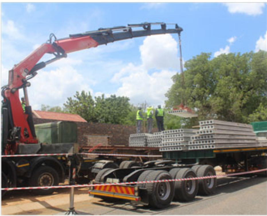
More than 40 tons of concrete elements were manufactured off-site and delivered to the construction site
